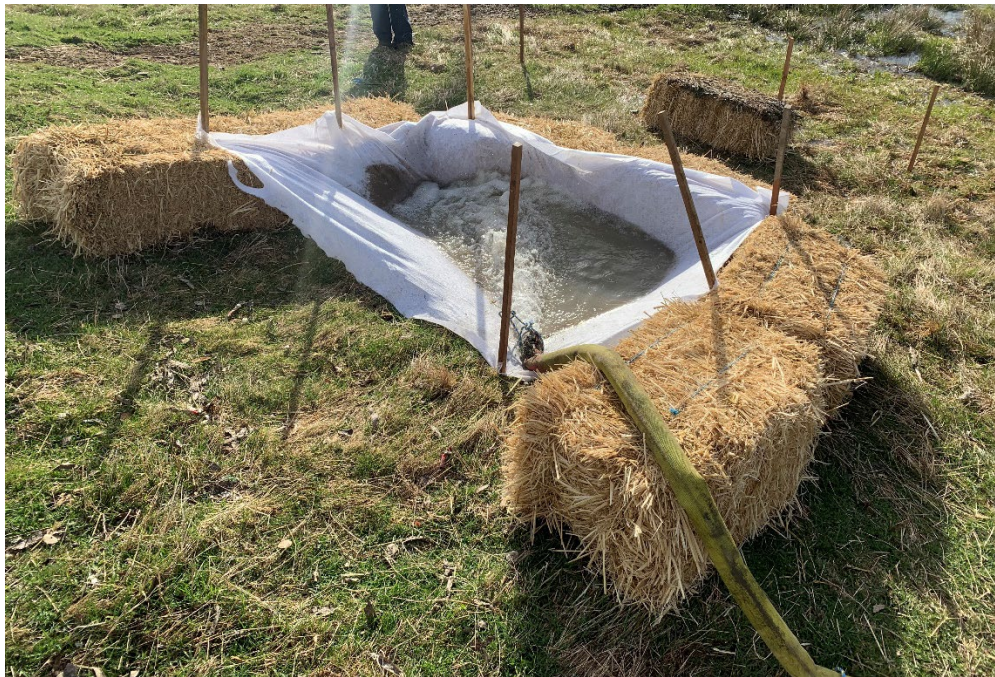
Figure 5: Standard Installation of Geofabric Filter Dam
